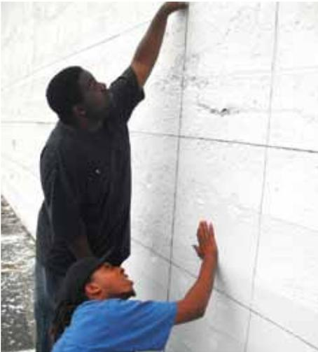
The grid lines must be straight, forming perfect squares. The best approach is to snap chalk lines directly on the wall.
